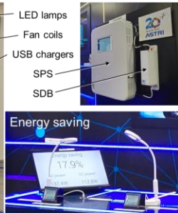
Fig. 9 DC power supply system installed at Hong Kong EMSD
