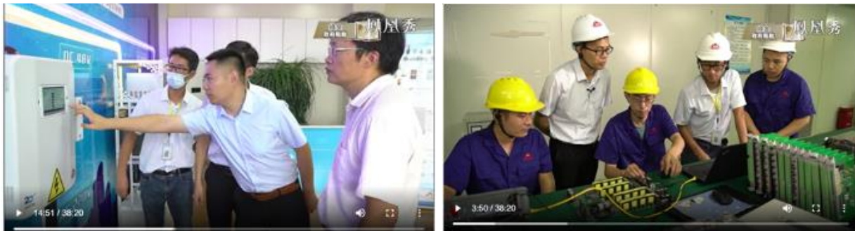
Fig. 8 DC power supply system installed at customer
